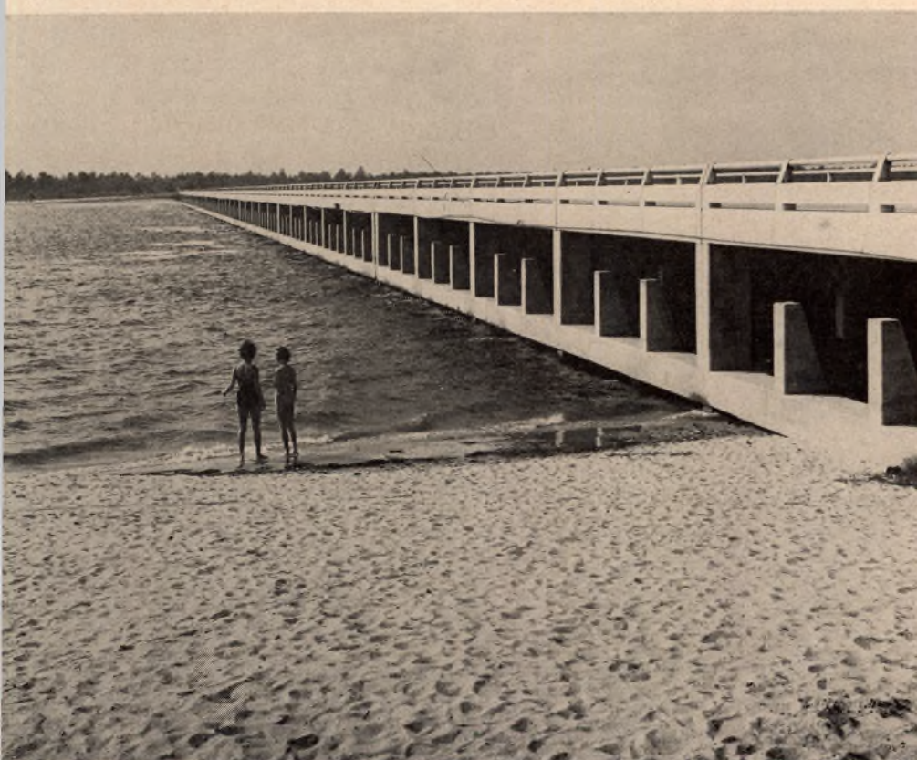
View of the new reservoir and spillway showing recreation area.
