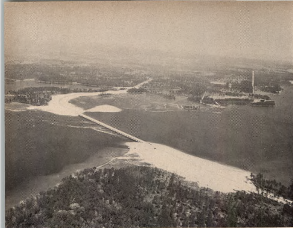
Aerial view of Deer Point Reservoir shows concrete spillway. In addition to carrying off the overflow, the spillway forms the base of a fine two-lane road.
